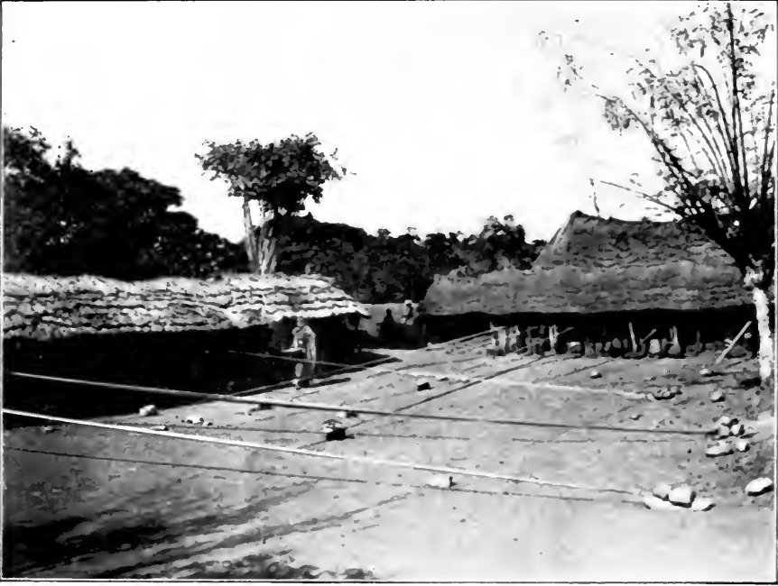
Transverse rope-walks in the compound.
